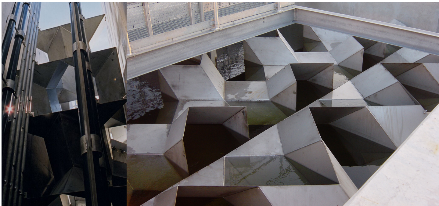
Channel Mixers installed on site at a UK Water Treatment works
